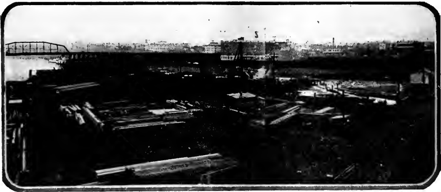
General view of the Supple & Ballin yard at Portland taken February 4, 1917, showing dredges and pile-drivers at work.
